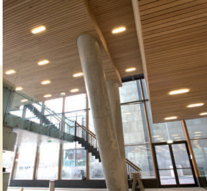
Above : Conservatorium Amsterdam, the Netherlands Architect: De Architecten Cie, Amsterdam Product : Linear open system 15 x 74 mm Wood : American Red Oak
