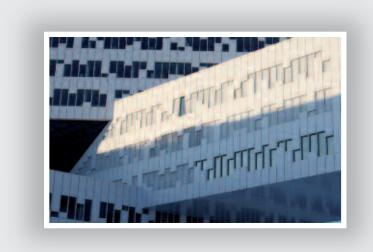
The new regional office of the Norwegian energy producer Statoil ASA, has a state of the art design. The highly energy efficient solution features a façade with prefabricated elements, integrated windows, insulation and solar-shading.
