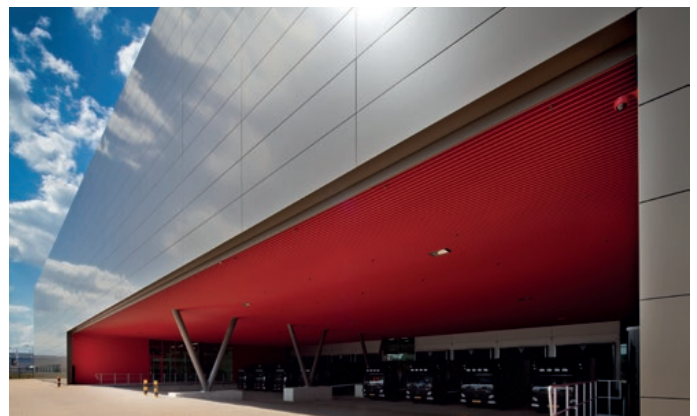
Above : Distributie Centrum The Sting, Tilburg, The Netherlands Architect: Van Oers Weijers Architecten Product : QuadroClad® QC300
