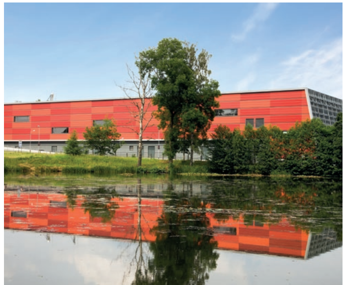
Above : Sunfilm Solar Factory, Großröhrsdorf, Germany Architect: IPRO Dresden Product : LinearClad™ F
