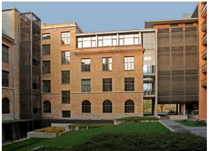
Above : Riverloft Apartments, Budapest, Hungary Architect : KÖZTI Architects & Engineer Product : 132S
